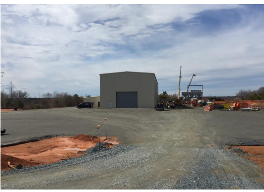
Smith-Carolina's new building going up
